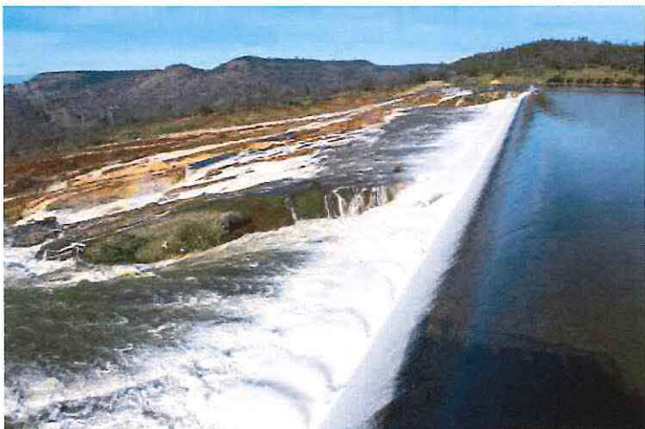
Water from the Oroville Dam Auxiliary Spillway at Lake Oroville flowed toward the diversion pool of the Feather River on Feb. 12, 2017. (Photo by Kelly M. Grow/ California Department of Water Resources.)
